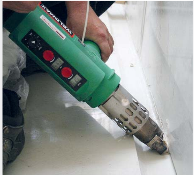
Extrusion welder WELDMAX working on a fillet weld seam.
