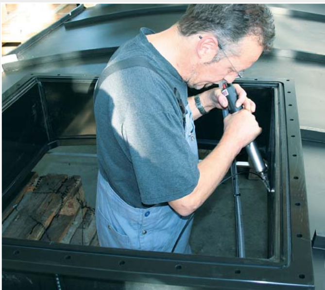
The inspection hatch is fixed with a DIODE S from Leister.
