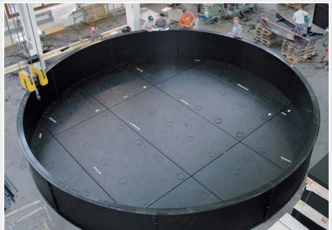
Checking the fit of the base elements and the lowest array of wall elements during fabrication.
