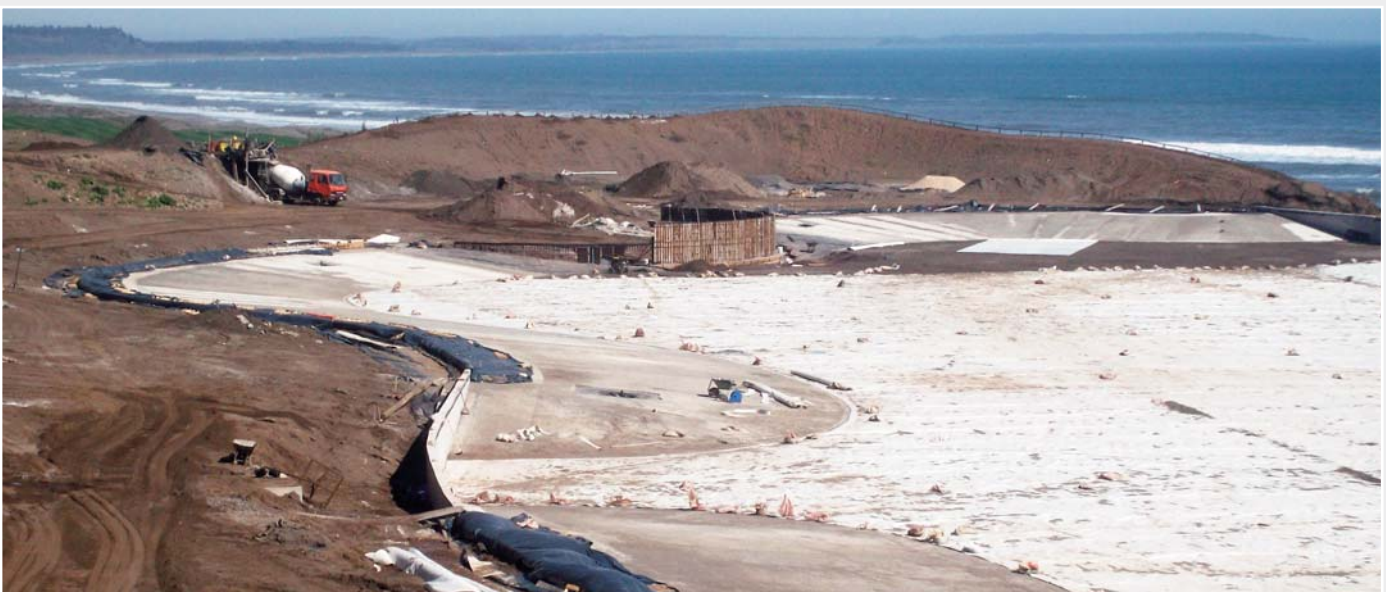
Las Brisas de Santo Domingo lagoon undergoing construction.
