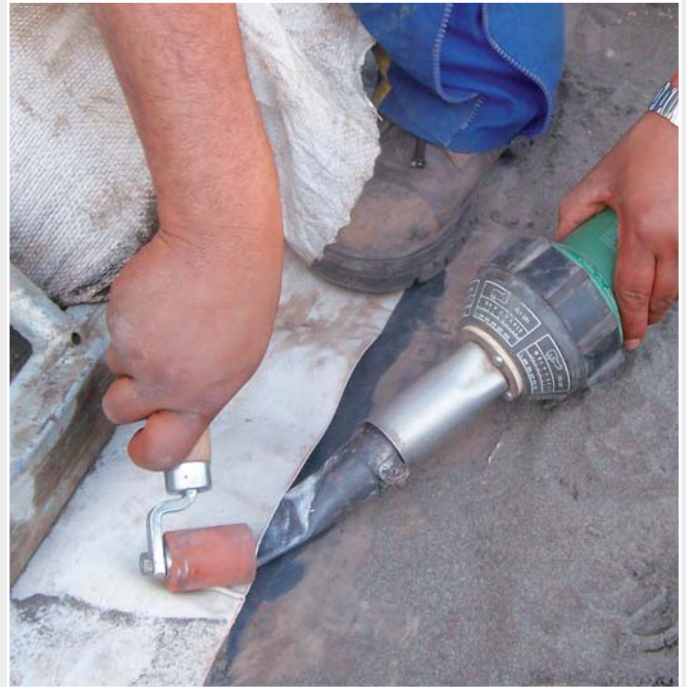
The proven manual welding unit TRIAC S for detailed work.
