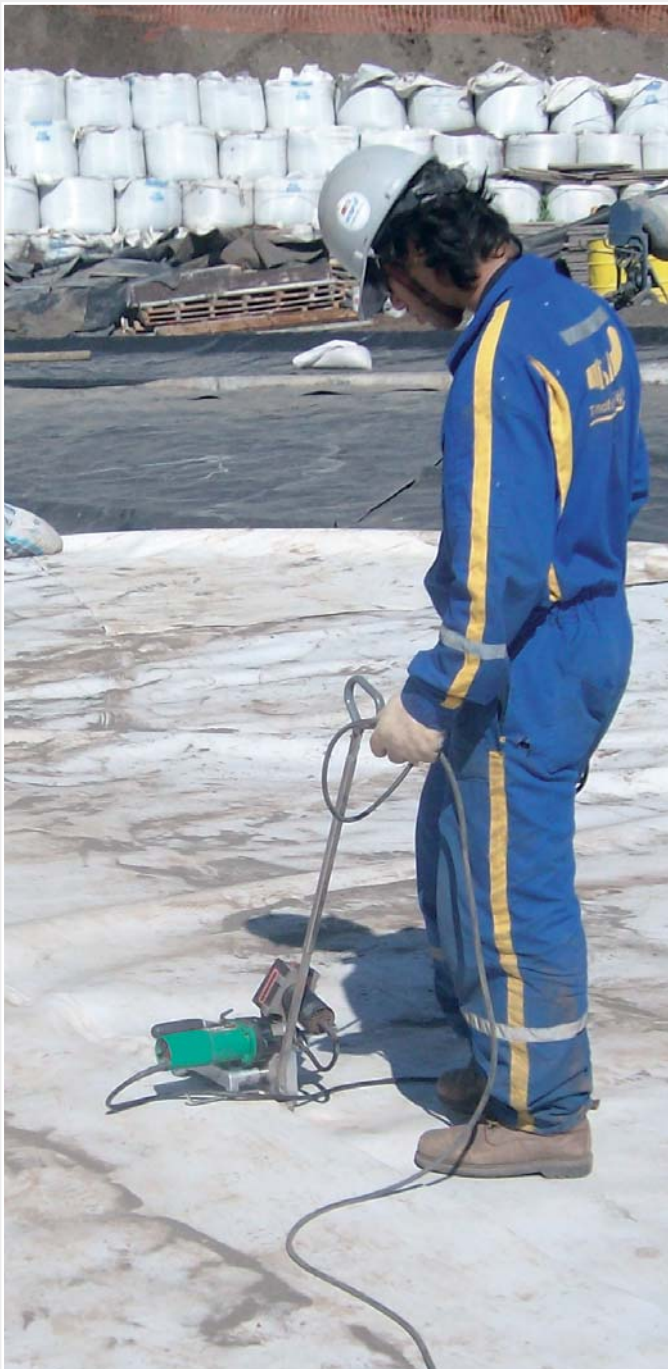
The compact and convenient TWINNY S with combi-wedge welding the uppermost layer.
