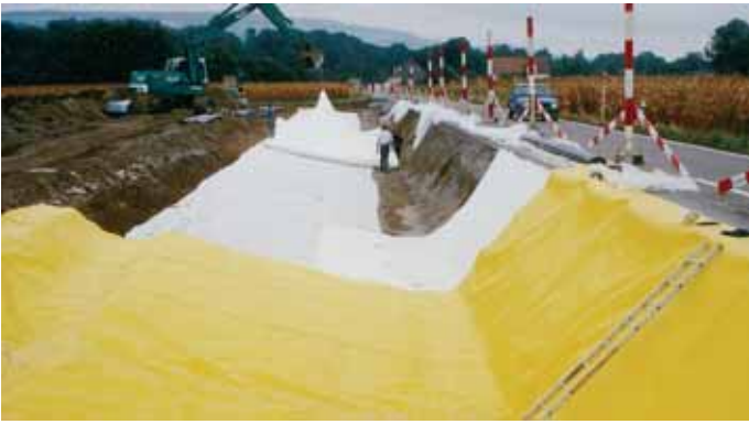
Geomembranes in road construction, Switzerland
