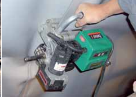
TWINNY T with combi-wedge, welding overhead in a tunnel.
