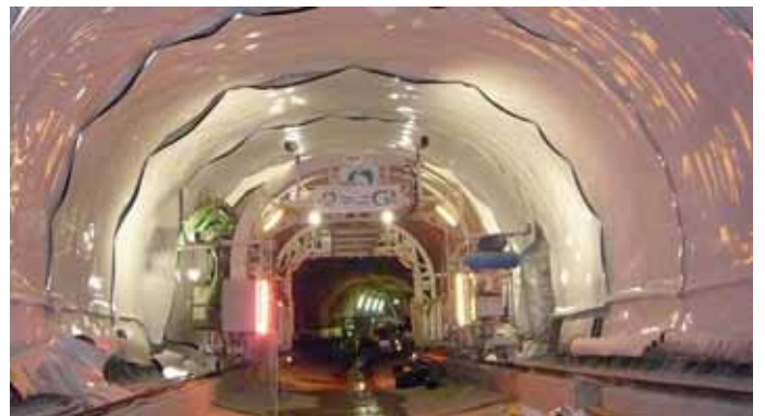
Tunnel construction in Germany
