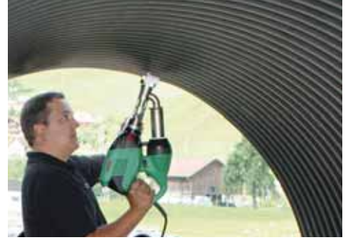
The handy WELDPLAST S2 welding vertically.
