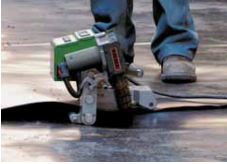
TWINNY T with combi-wedge used to weld a HD-PE liner.
