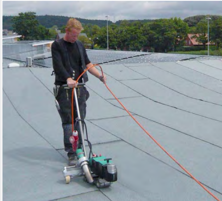
2. Single layer system: Quickly and easily welded with high quality results.
