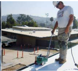
Work doesn't stop at the edging boards.
